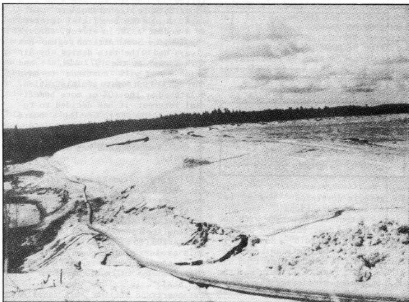
Part of the huge tailings dam at Elliot Lake: this waste contains up to 90% of the radioactivity of the original uranium
